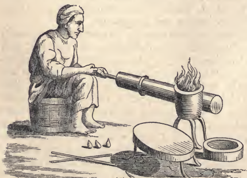
No. 113. Chinese Single Bellows, and Tinker.
